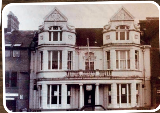
Chard Working Men's Club (Now Flats)
