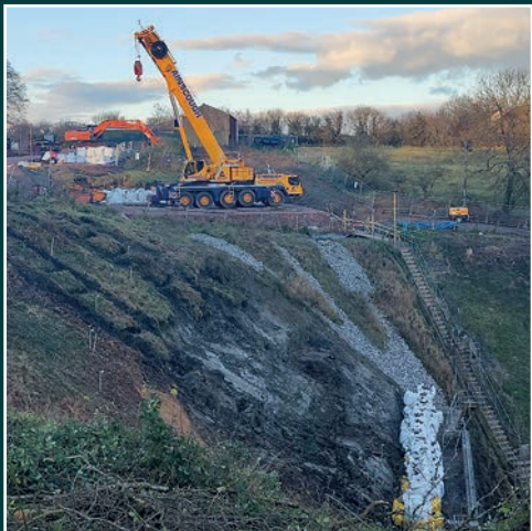
Railway embankment stabilisation nearing completion 10 February 2024
